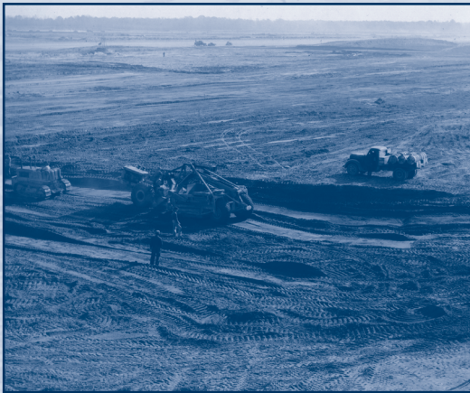
View illustrating the magnitude of earth moving required to construct the runways.
